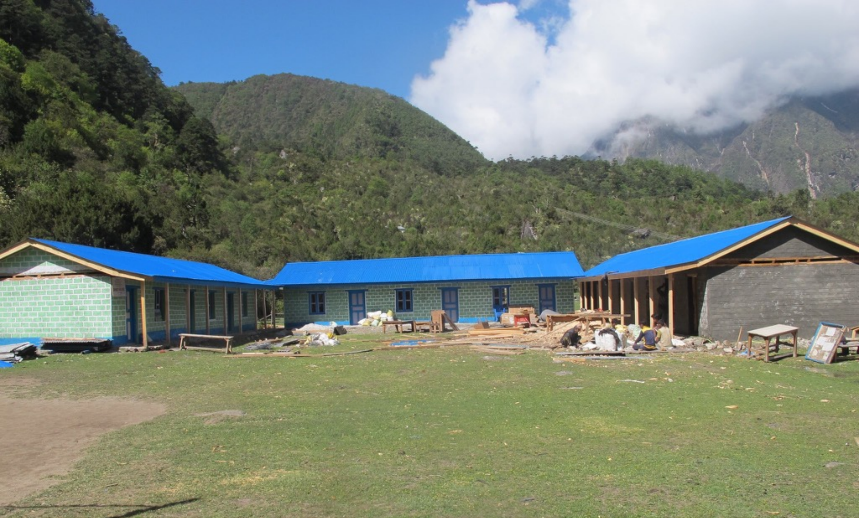
Ghunsa School - Kanchenjunga region totally rebuilt July 2015
